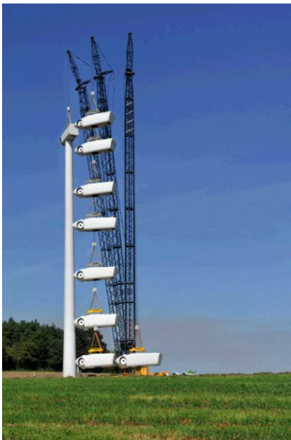
Source photo : Q ENERGY France
