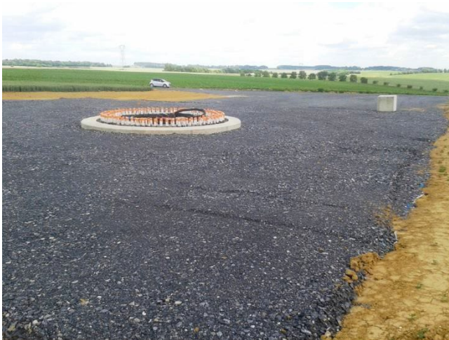
Source photo : Q ENERGY France
