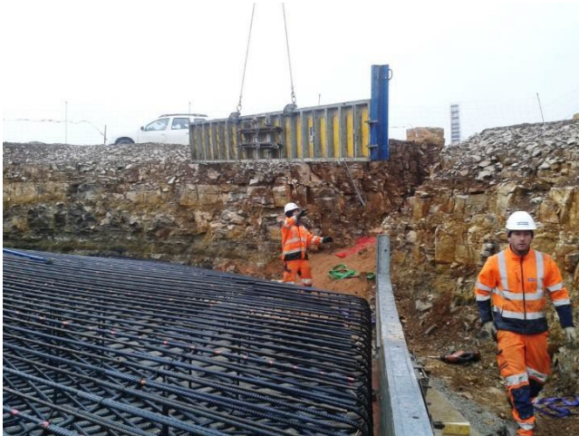
Source photo : Q ENERGY France
